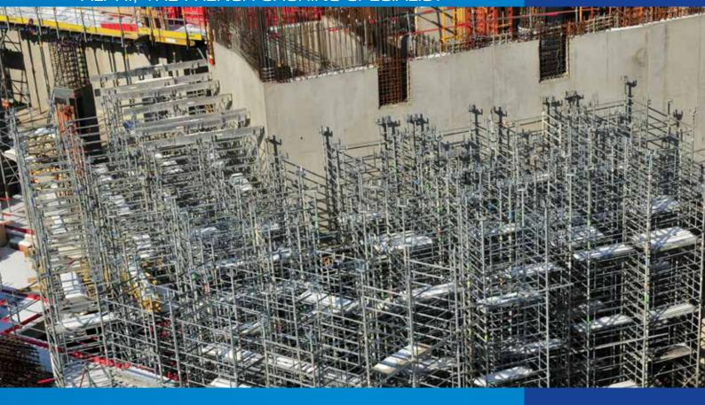
The A120 tower is a shoring tower that can be assembled and disassembled in complete safety. High-performance, it allows a load of 3 tonnes/foot.
